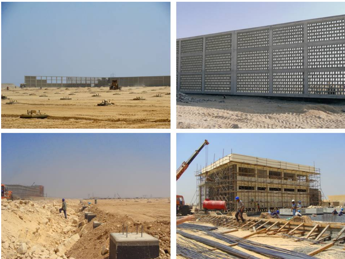
Figure 6-1 Progress of Solar Island Civil Works
