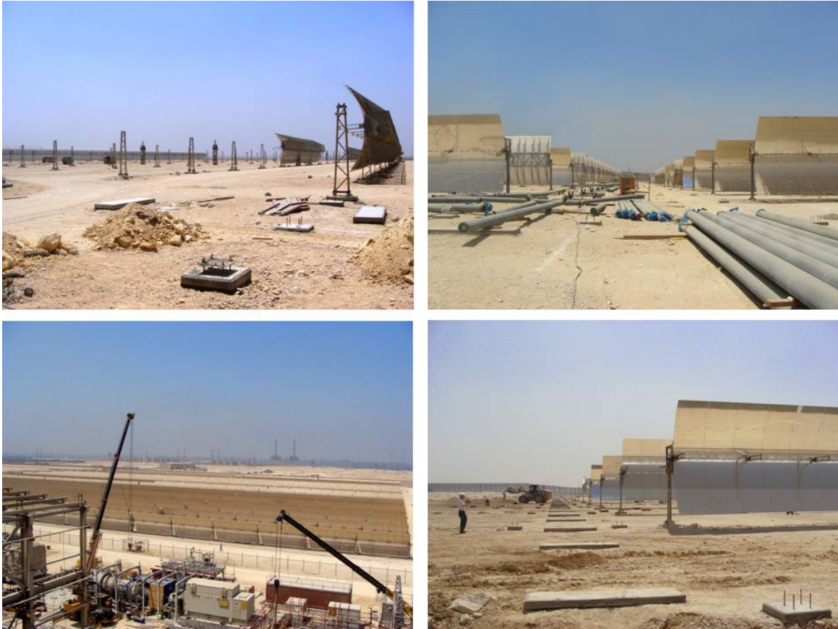
Figure 6-2 Collector Installation Progress
