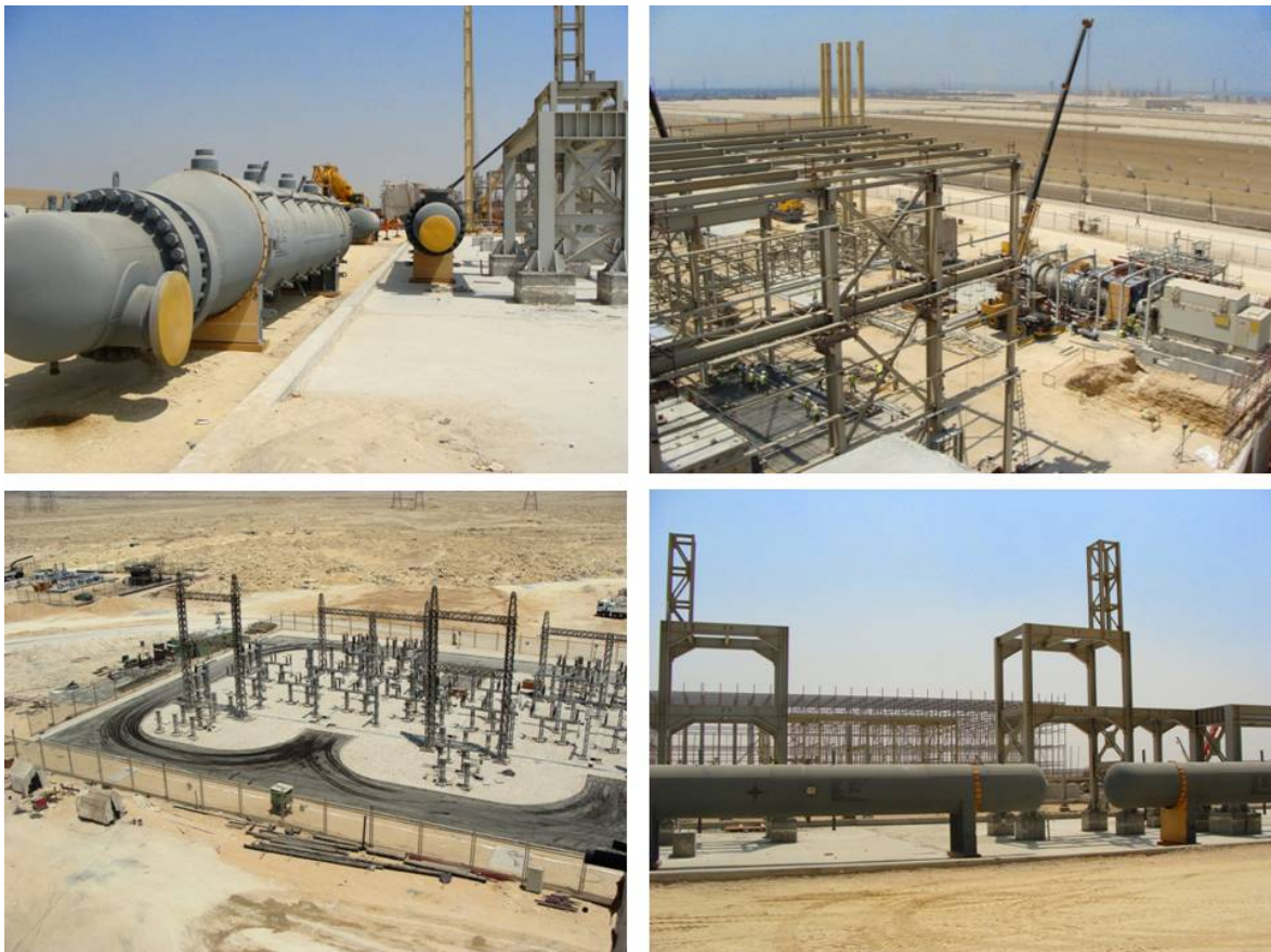
Figure 6-3 Civil and Mechanical Works Progress of Combined Cycle
